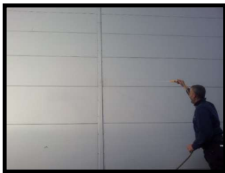
Water testing of the architectural wall panels
